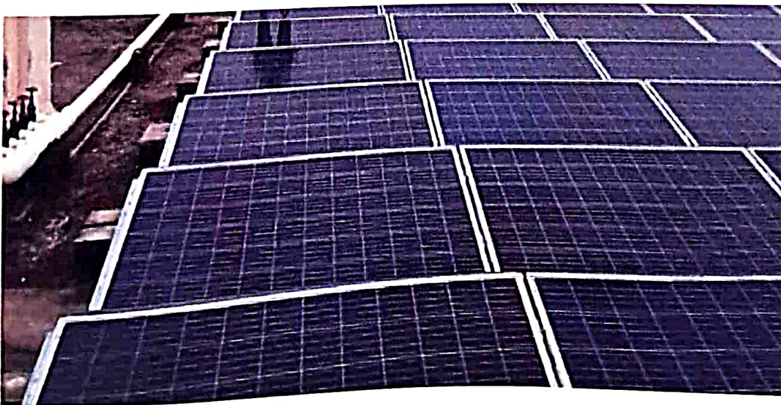
SOLAR PANEL INSTALLED IN ROOF TOP
